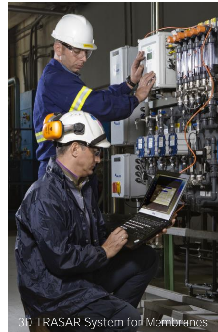
Reverse Osmosis System
